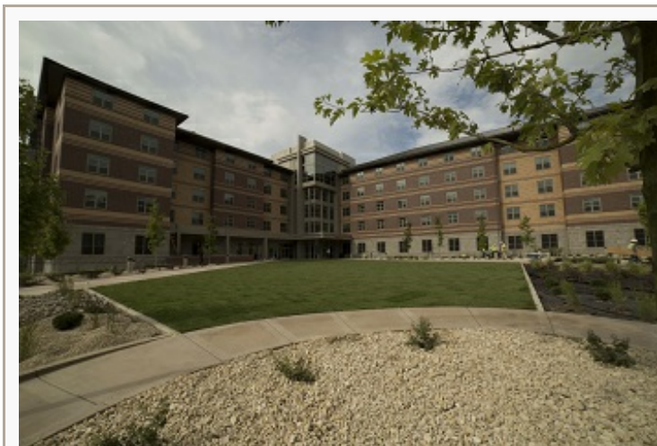
Construction workers put the finishing touches on Peavine Hall, the University's newest residential hall scheduled to open Aug. 13 with a free public viewing. Photo credit: Robie Aker.
