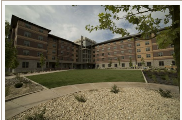
Construction workers put the finishing touches on Peavine Hall, the University's newest residential hall scheduled to open Aug. 13 with a free public viewing. Photo by Robie Aker, University of Nevada, Reno.
